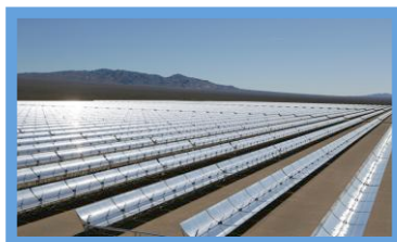
Project Name: Nevada Solar One Developer: Acciona Electricity Purchaser: NV Energy Location: Boulder City, Nev. Technology: Trough Capacity: 64 MW Source: Acciona North America
