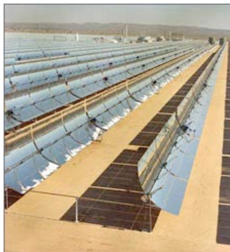
Figure A-2. Parabolic Trough Solar Thermal Power Plant, Kramer Junction, California (Source: National Renewable Energy Laboratory)
