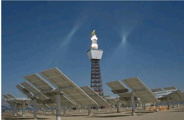
Figure A-4. 10 MW Solar Two Power Tower Plant, Daggett, California (Source: Sandia National Laboratories)
