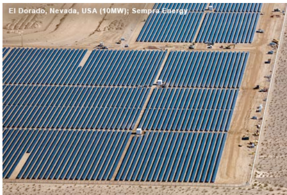
Figure A-7. 10 MW Large-Scale Thin Film Photovoltaic Power Plant, El Dorado, Nevada (Photo: Courtesy of First Solar)
